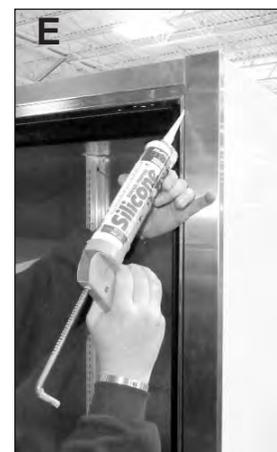
**E.** Reinstall the J-strip with the screws and apply a new bead of clear silicone to seal the J-strip to the edge trim.
