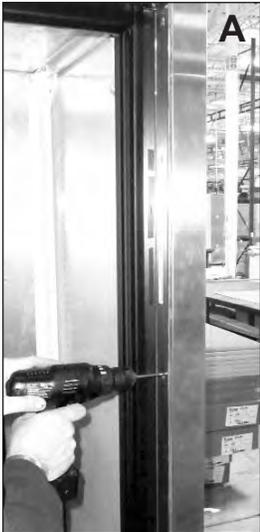
**A.** Back-out and retain the frame screws that secure the “J”-strip that covers the inside edge of the trim piece. If the door hinges on the side of the edge trim that needs replaced, it will be in the way of the frame screws, and will need to be removed first in order to access the screws.
