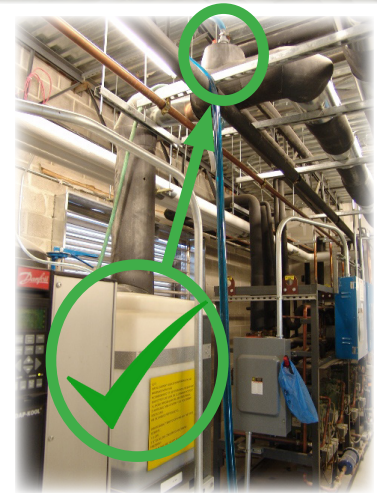
Needed vent properly installed
