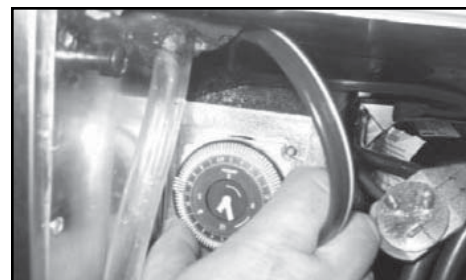
Image 4 (Defrost timer on TSID and TDBD-36/48 models).
