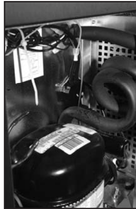
Placement of Relay (above compressor)
