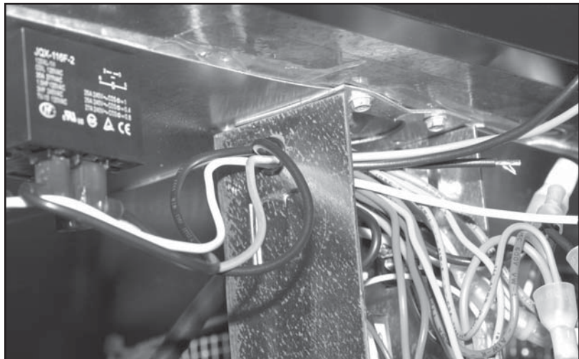
Figure 7. Routing relay wires
