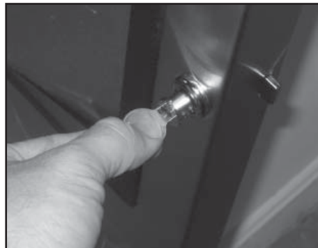
Image 3 (Removing plug / key receptacle)
