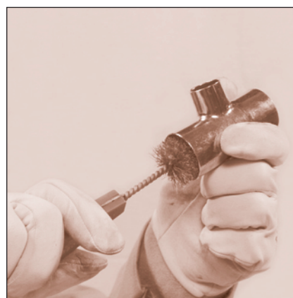
FIGURE 17: Cleaning: Fitting brush
