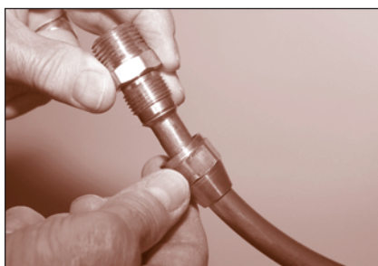
FIGURE 28: Flare fitting/flared joint during assembly
